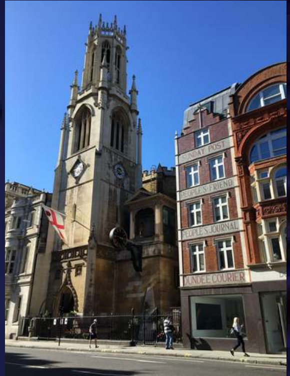
The building to the right (with Dundee Courier on it) is 186 Fleet Street- the fictional site of Sweeney Todd's barber shop. Next to it is St Dunstan's Church
